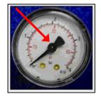
This picture shows the needle on zero, which will cause problems with the boiler's normal operation. Ideally when the boiler is cold the needle should read 1.5bar (indicated by the arrow). When the boiler is in operation it's normal to see the needle rise to about 2.5bar.
