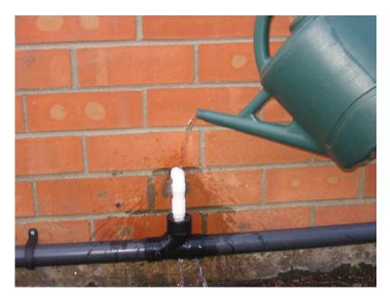
**Note 3** — You should not attempt to thaw a condensate drain pipe if you cannot easily reach it from ground level. Be aware that any water used can quickly freeze if it falls onto pathways – causing a possible slip hazard.
